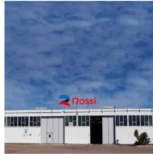
Planetary Division facilities Lecce - Italy
